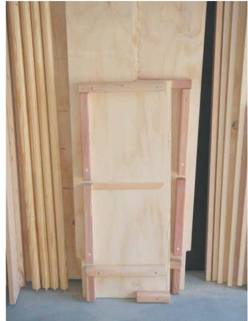
The two side panels, showing how the  $1\frac{1}{4}$ " x  $1\frac{1}{4}$ " 'ribs' have been permanently attached.
