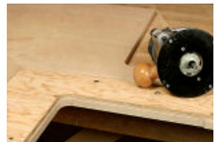
The final, trimmed edge (on the inside of the three-sided infill frame) is produced using the master template and the same router, guide and bit combination that made the initial cutout.
