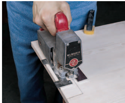
Figure 2: Use a jigsaw to notch the counter so it fits between the cupboard sides (see the Counter drawing at right for dimensions).
