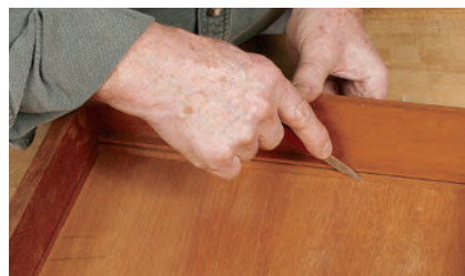
To create the second tongue on the drawer bottom, establish the shoulder with a knife line. Cut all tongues with a shoulder plane.
