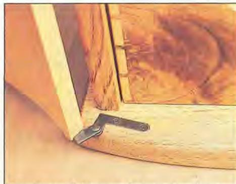
**Photo D:** Attach hinges to door, position door on cabinet, align both hinge leaves, and mark hinge location on the top and base. Then, cut cabinet gains as shown.
