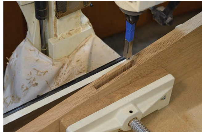
A 3/8 " mortising chisel creates a mortise in each leg. Since the leg's reference edge on top is already angled, the depth stop won't work. Wrap a piece of painter's tape around the chisel to indicate the required depth.
