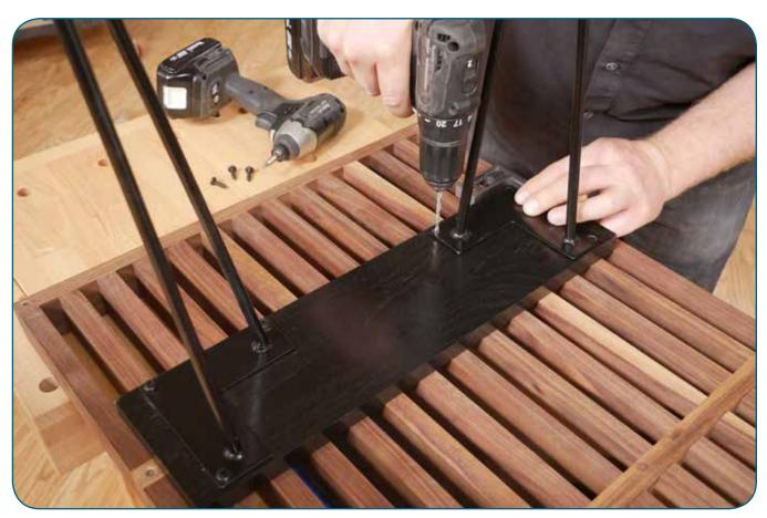
Cut and sand a wood cleat. Color it black with dye stain and apply a topcoat after the stain is dry. Attach the cleat to the top, and screw the I-Semble Hairpin Table Legs to the cleat with the screws included with the hardware.
