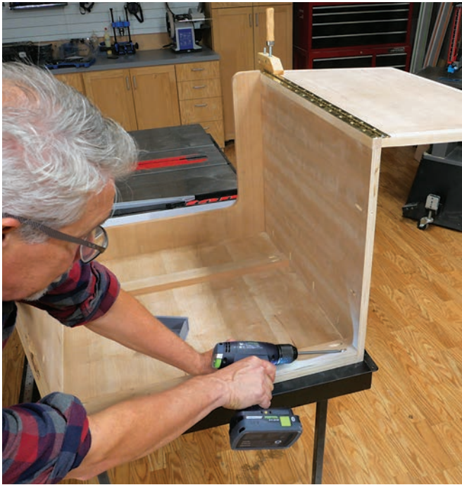
Install a pair of plywood lift supports inside the cabinet (left). Then attach the sewing machine lift hardware to the supports (right). The lift is adjustable to accommodate almost all sewing machines. Here the cabinet's top work surface is removed for clarity.
