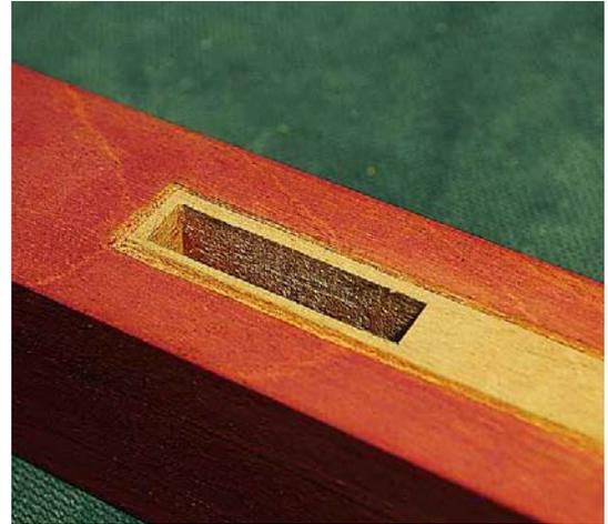
Figure 1: Slice tiny v-channels around the perimeter of the joint areas with a sharp chisel or utility knife to help prevent glue squeeze out from smudging the dye.
