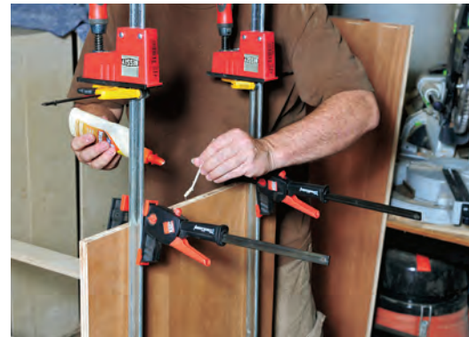
Glue is applied into the biscuit slots (and onto the biscuits themselves) using a pipe cleaner [chenille stem] with its end bent into a "U."
