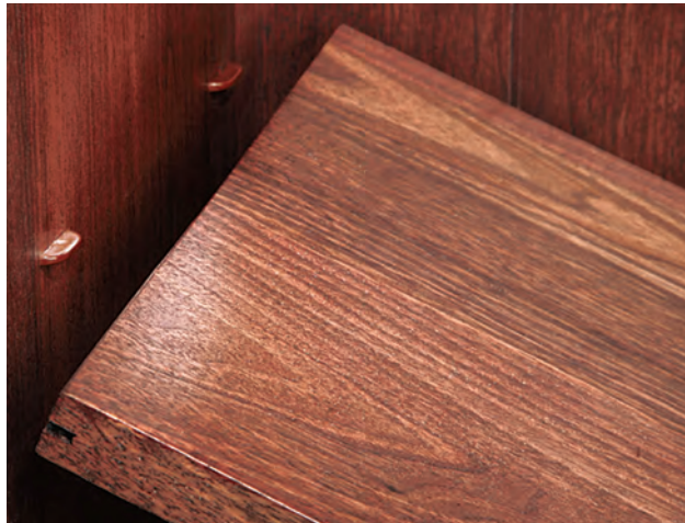
Red mahogany oil stain (left) added colorful highlights to the walnut lumber — popping the grain nicely. Above, the ends of the shelf (turned around so you can see the back) have a groove sliced into them that slides over the winged shelf pins.
