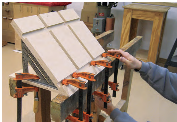
Glue and clamp the table to the base. Clamp a speed square at one or both ends to ensure the table is set at exactly 45° relative to the base.
