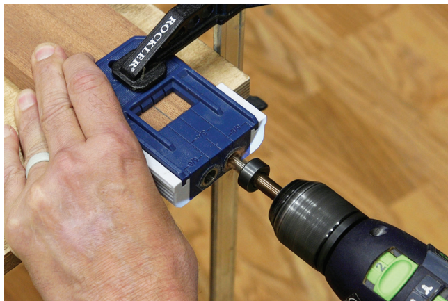
The stiles and rails of the door are joined together with 3/8"-diameter dowels. Square ends on each piece of the door frame are critical to its assembly. They form a frame on which the hinges will be mounted.
