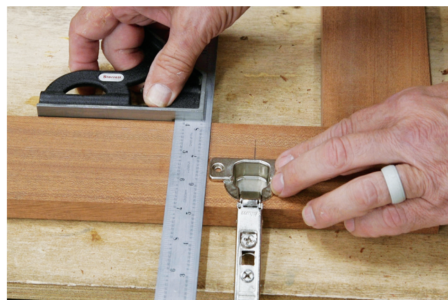
With the holes bored, mount the hinge cups to the door frame with two screws. Check with a square to ensure that you have the hinge cups properly aligned. Use a self-centering drill bit to bore the screw pilot holes.
