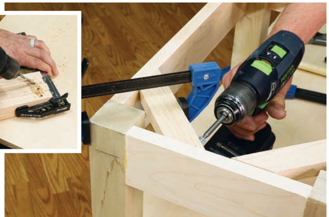
Photo 12: Drill holes into the angle braces as shown in the inset photo. Clamp an angle brace into place and then drive 1\frac{1}{4} "-long panhead screws into the aprons. Attach all four angle braces.
