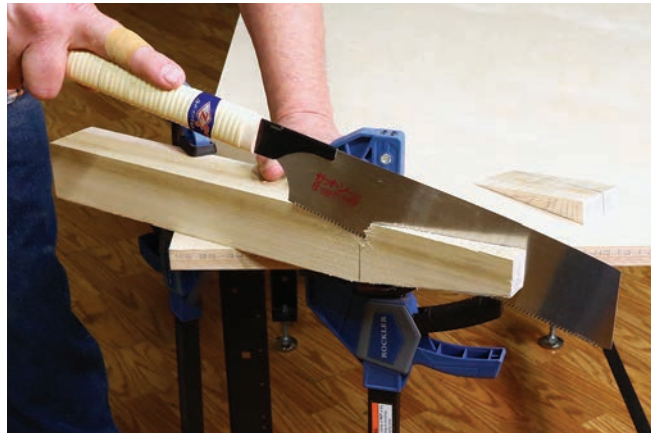
Photo 2: Mark out the same angle on an adjoining face of the leg. Remove that triangular section. Now the leg has a 1\frac{1}{8} "-square "foot" and two adjoining angled faces, called tapers.
